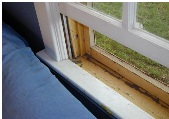
Figure 6. Picture of an old window with deteriorating lead-based paint in the window trough
